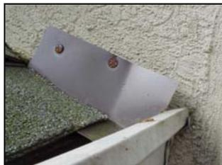
A functional kickout flashing can NOT be mounted on top of the cladding.
