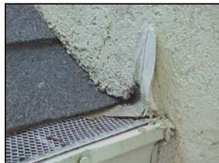
Hand or field made kickouts fail at a very high rate.
