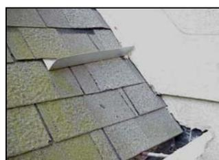
Diverter flashing is NOT a substitute for a kickout flashing.
